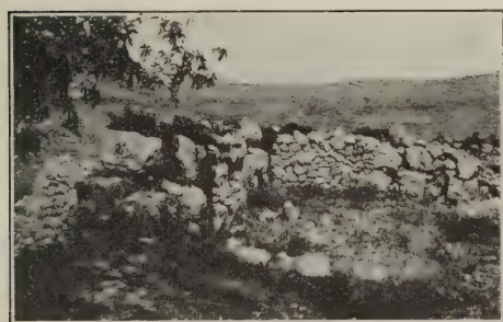
12. North wall of north tower
